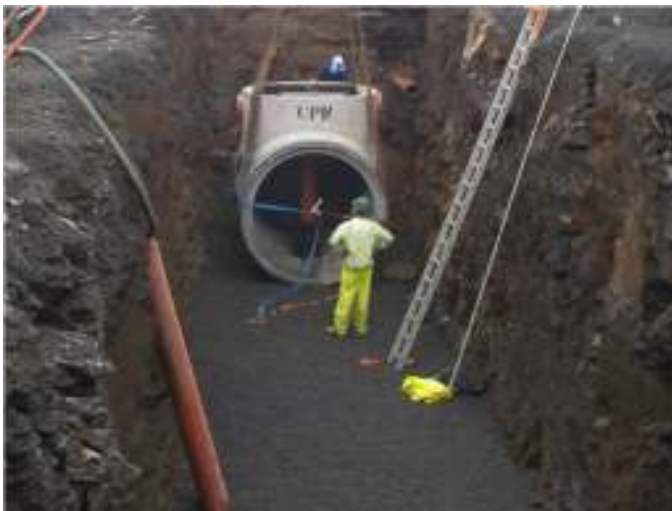
IRM-10 C-Class, Trident 5000 Regenwaterfilter in 60.000 L tank
