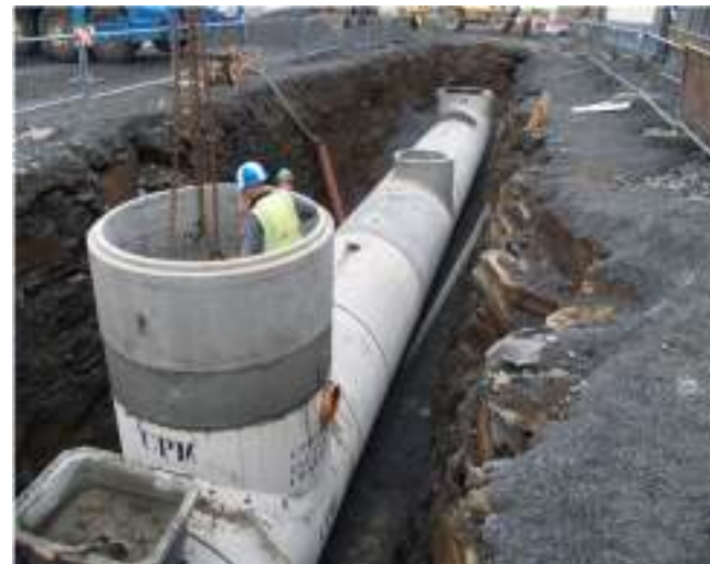
IRM-10 C-Class, Trident 5000 Regenwaterfilter in 60.000 L tank
